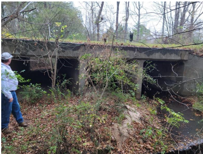
Dried Indian Creek on E. Soule Street - 9'x6' Triple Boxed Concrete Culvert that is approximately 11 year's old. The County does not feel it would support the weight for commercial/industrial development that is contemplated near this site.
